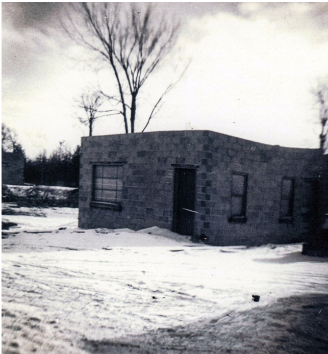
Sanford Post Office under construction in 1946. Edwin O. Hess was postmaster. This was the first “stand alone” building built to house the Sanford Post Office. In this building today is the business of The Beach Tanning Salon. Photo from the Sanford Historical Society collection.
